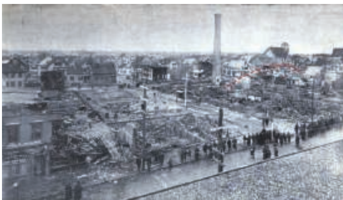
FIGURE 1. The aftermath of the 1905 explosion and fire at the R.B. Grover Shoe Factory in Brockton, Mass. The trajectory of the boiler is shown as the red arc
